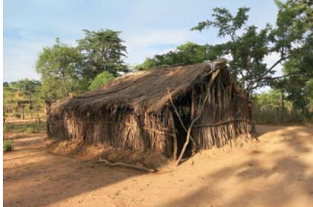
Left: BEFORE MARANATHA: Adventists in Kainja built their first church out of materials at their disposal: dried sunflower stalks and sun-dried mud “bricks.” Right: READY FOR WALLS: Adventists in Kainja have been baking bricks for walls. The weather-proof roof means their walls will last for years.
